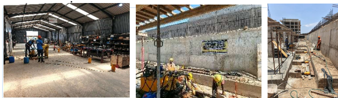
Figure: Testing and installation of large structure elements
