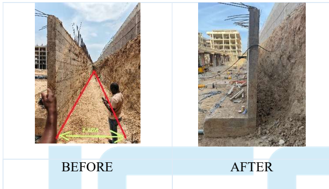
.Figure: Proper alignment of the wall.
